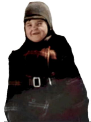
Little Jackie playing outdoors after the Blizzard of 1936 at the Villa Ave house in Buffalo.
